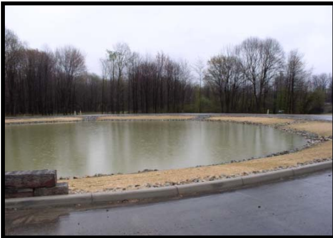
Typical Retention Basin
